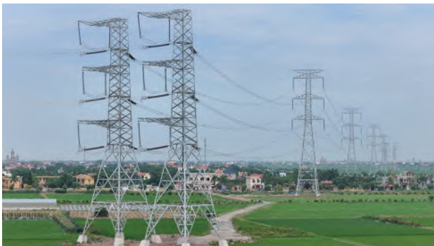
The 500kV circuit-3 transmission line, Nam Dinh I TPP - Pho Noi section was completed and energized on the afternoon of August 19 th 2024
