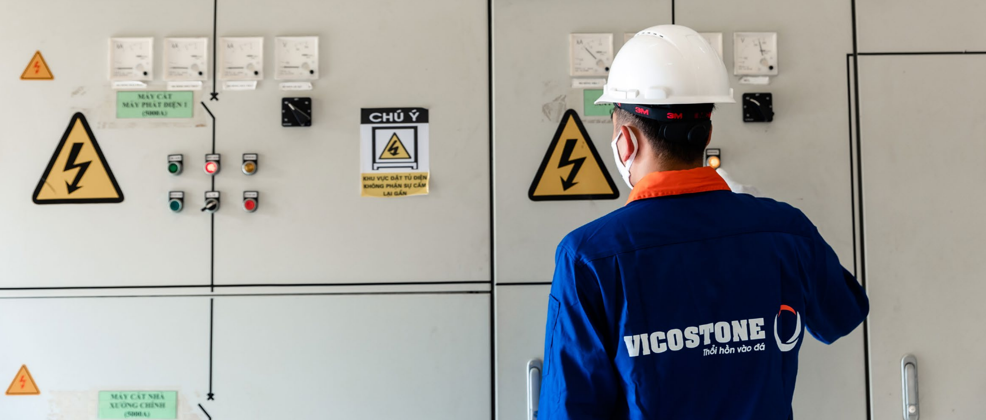
Total energy consumption at Vicostone's parent company in 2023 (Jun):
